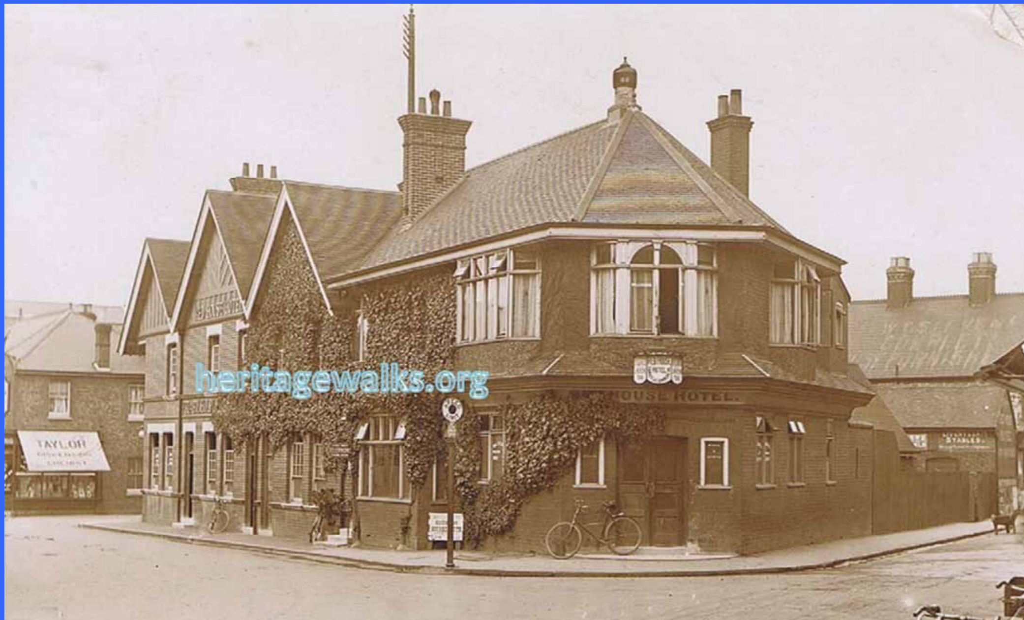
In 1890 the Red House in Woking was letting their waste flow into the street.
