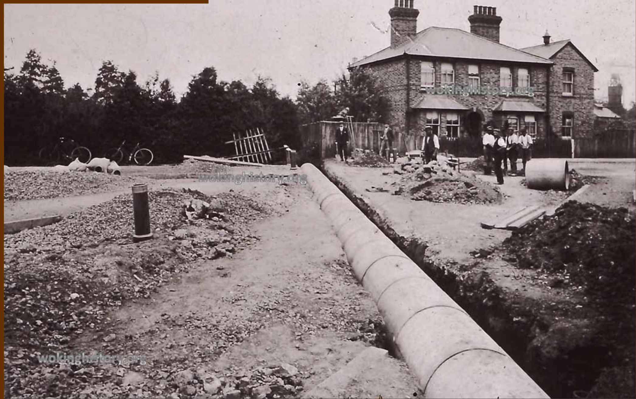
Pipes being laid under Courtney Road show that some progress was being made in the mid 1890's.
