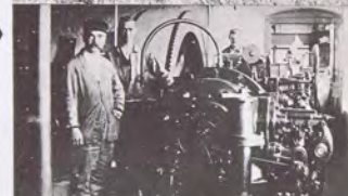
The old Crossley twin-cylinder engine in the engineers' shop (Mr T. Jordan senior, then Maintenance Overseer, on the left)
