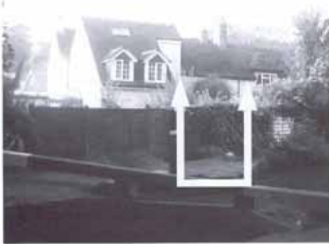
The Lock-keeper's Cottage, showing the original section between the two arows.
