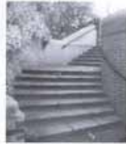
The steps up to the road at Kiln Bridge.
