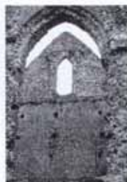
Looking through the 'right-stair' into the South Transept
