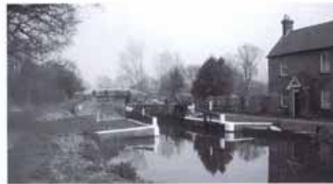
The turf sides of Walsham Gates, with the lock-keeper's cottage on the right.
