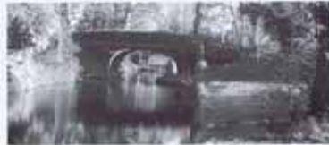
Scotland Bridge - one of the few 'original' arches on the canal in this area.
