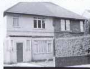
H.G. Wells' house in Maybury Road. Look at the house next door for a better idea of how Wells would have seen his house.
