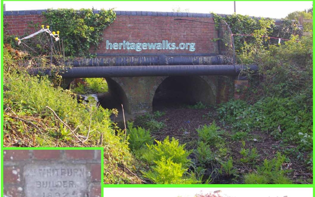
he new bridge over the Hoe Stream at Elmbridge is just the latest in a long line of bridges on that site. The one shown here was built in 1892 by a local builder called James Whitburn (a stone on the downstream side used to proudly proclaim his name). He was paid £670 by Guildford Rural Highways Board to replace the old wooden bridge that was only 12ft wide and evidently falling apart.
