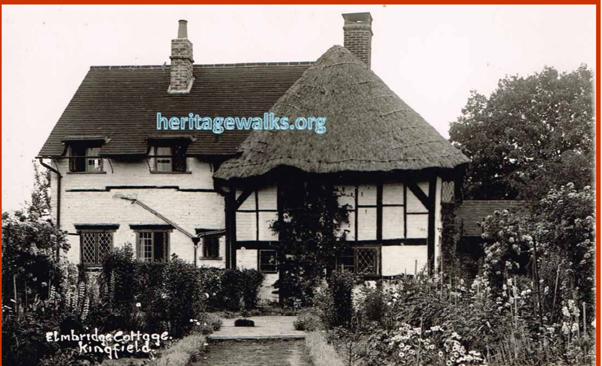
The thatched Elmbriidge Cottage in Kingfield Road has signs of an internal jetty over its open hall.
