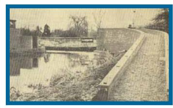
Construction of the new bridge took just a few months with the ramps on either side constructed first. By March they were ready to receive the new six-ton steel bridge that was capable of being swung on the Horsell side of the waterway - should any barge venture up this part of the canal. It was finally opened on the 17th May 1960 by Horsell Councillor, Archie Benstead (accompanied by a number of other councillors and officials).
