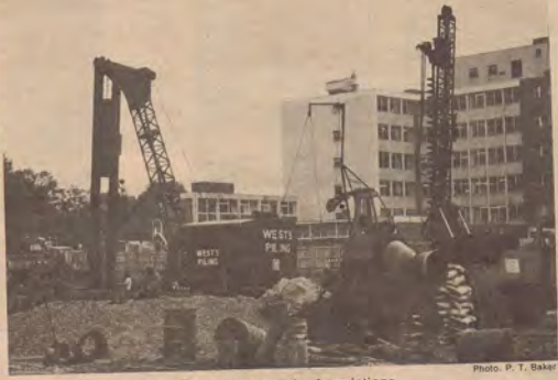
Work starts on the foundations.
