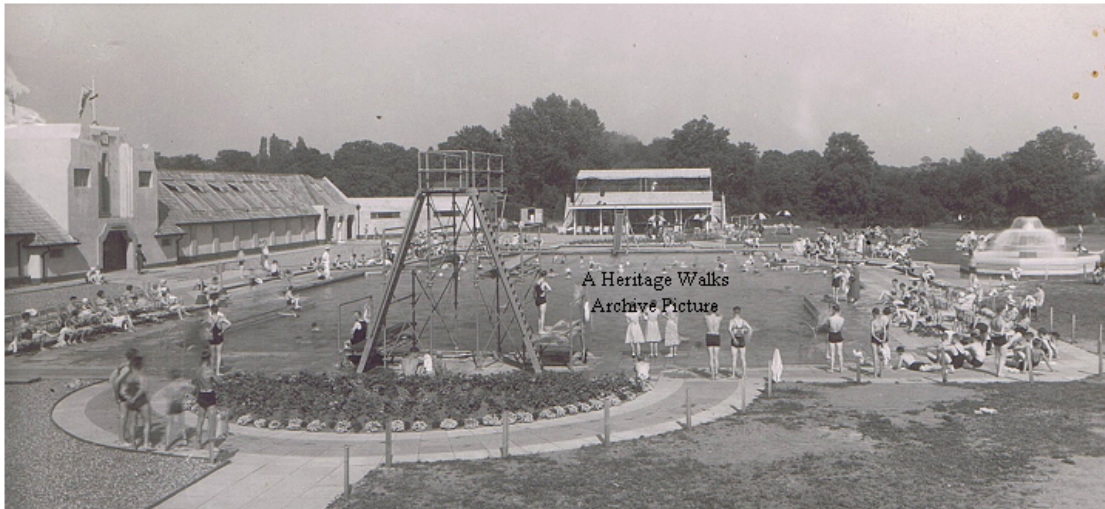
The 1930's Outdoor Swimming Pool in Woking Park was said to 'float' on the refuse of the former dump on the site.
