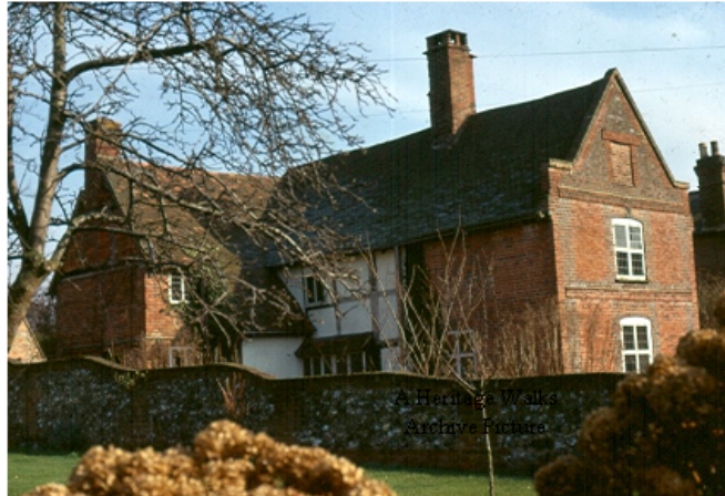
One of the oldest houses in Horsell is Esgairs on Horsell High Street. It dates back to the late 15 th or early 16 th century and is a grade II listed building.
