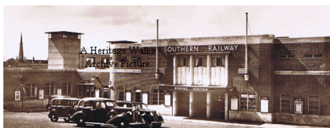
The main station entrance to the south was rebuilt in the mid-1930's in what has often been described as the 'Southern Railway 'Odeon' Style'.
