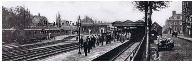
The original station at Woking can be seen in this photograph taken from where the buses now stop in The Broadway. The line in the foreground has been removed and what was then platform two is now platform one.
