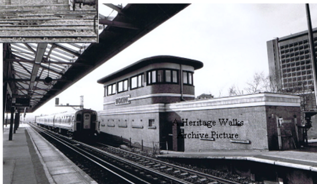
There were at one stage three signal boxes around Woking Station (including the Woking Junction box, pictured above left), with others at Maybury and Goldsworth. All were replaced in 1937 when the new signal box (now a Grade II listed building) was built as part of the electrification of the main line through Woking.
