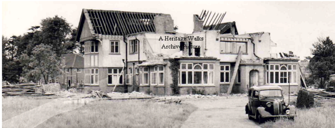
The Royston Chase Hotel being demolished in 1957
