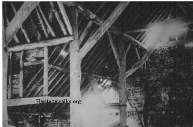
When the Palace was abandoned in the 17 th century part of the palace complex became the outbuildings to Woking Park Farm. One of the old halls became a barn, pictured here in the 1940's before it too collapsed.
